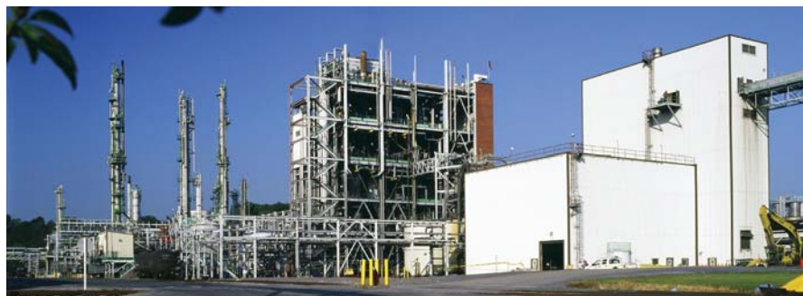
1. First in the U.S. In 1983, Eastman Chemical Co. put the first commercial coal gasification facility in the U.S. into service in Kingsport, Tenn. The open structure in the middle houses the gasifier block, and the white building to the right contains the rod mills that grind its coal input. On the left and in the background are the plant's acid gas-removal columns. Courtesy: Eastman Chemical Co.
