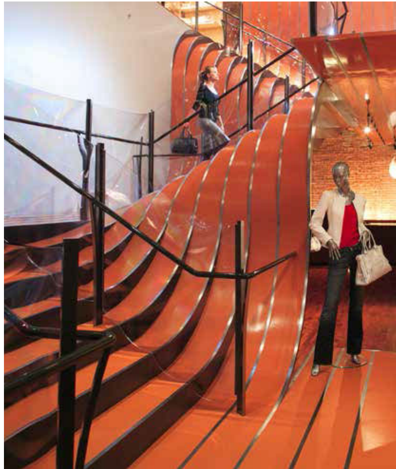
Eastman Spectar™ copolyester offered the formability, durability, and reflectivity Heatherwick's vision required for the balustrades.
