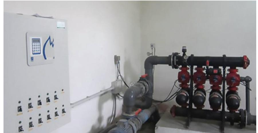
Central control unit to program irrigation time and flow
