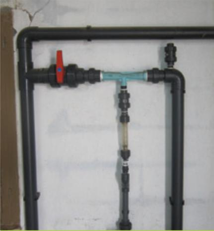
When there is no injection pump available, the product can be incorporated into the water by suction through a Venturi system
