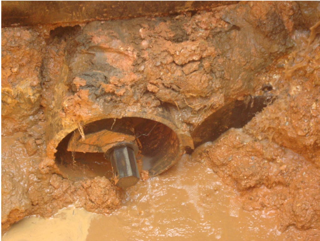
Photo 5: Boring equipment breakthrough in receiving pit.
