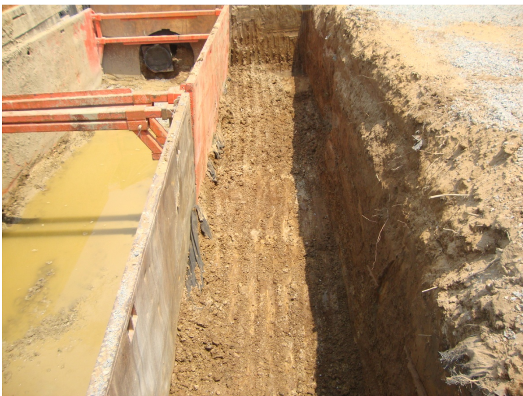
Photo 4: Preparation of receiving pit for 30" casing bore.
