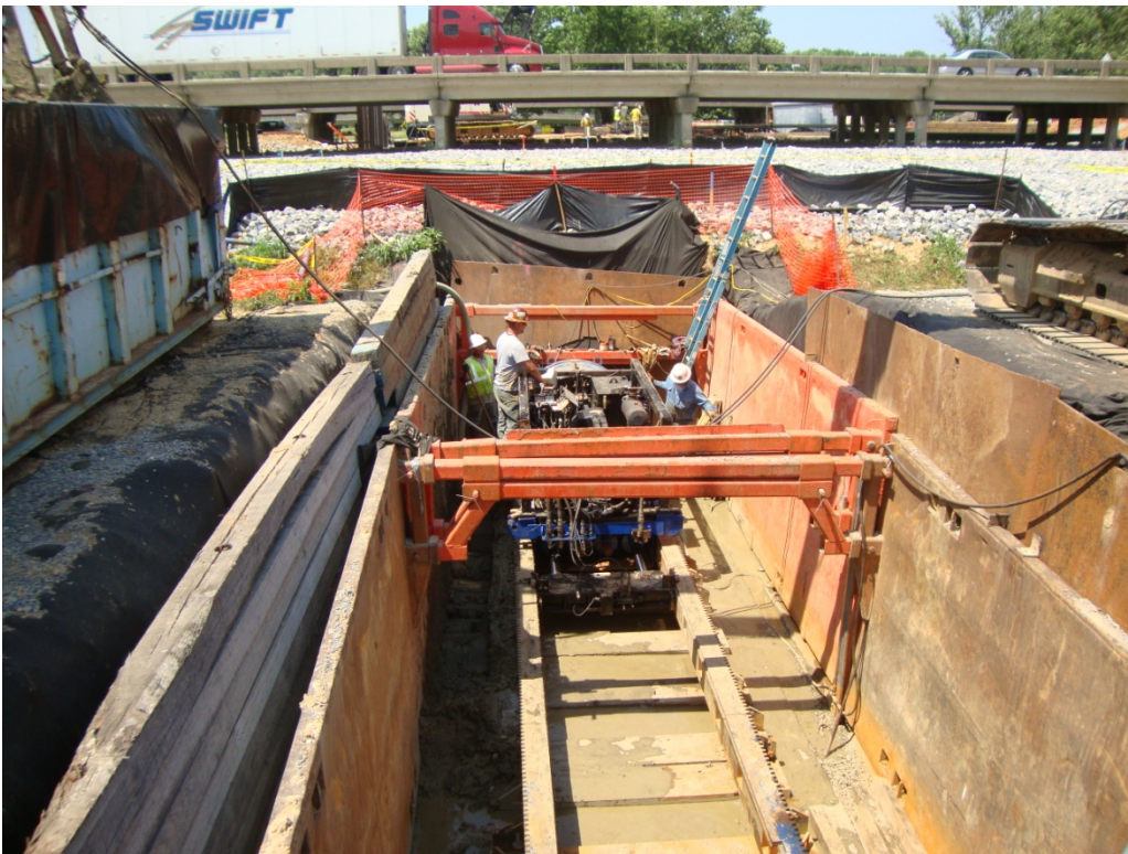
Photo 2: Boring equipment set in jacking pit looking north toward I-20.
