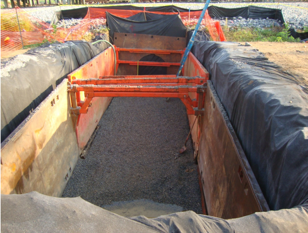
Photo 1: Bedding stone in place in jacking pit looking north toward I-20.
