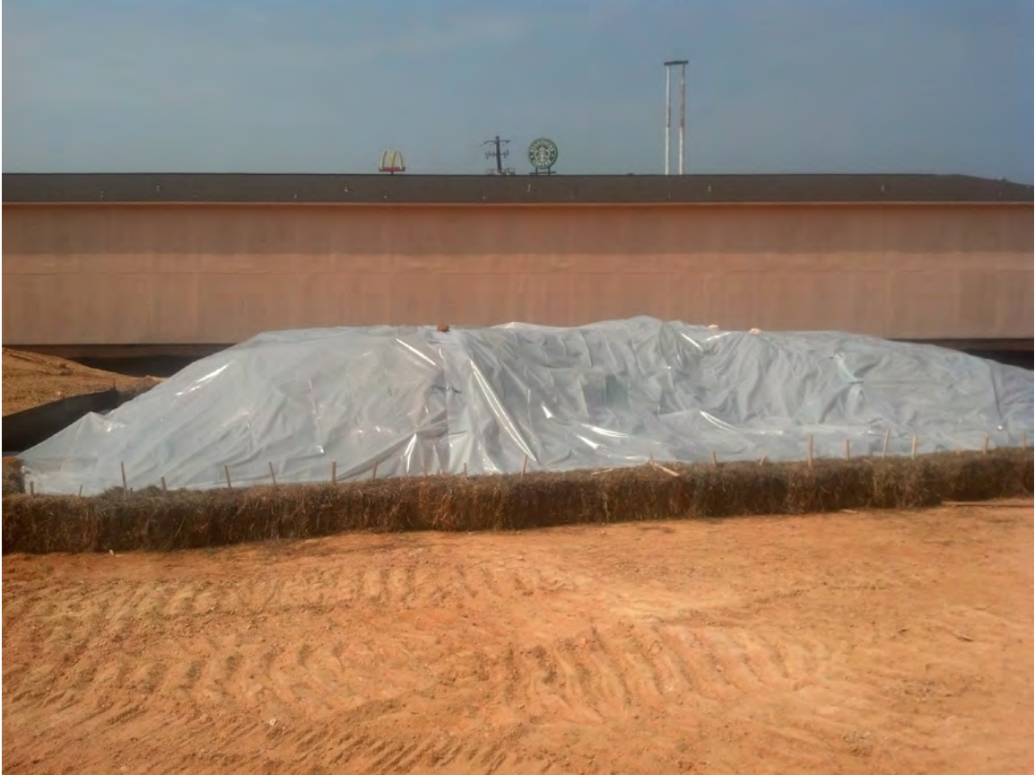
Photo 5: Temporary staging of PCB-containing soil (greater than 1 and less than 50 ppm) covered by 6 millimeter plastic sheeting and surrounded by silt fence and hay bales.
