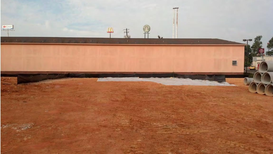
Photo 3: Construction of temporary staging pad. 6 millimeter plastic sheeting is visible in the background.
