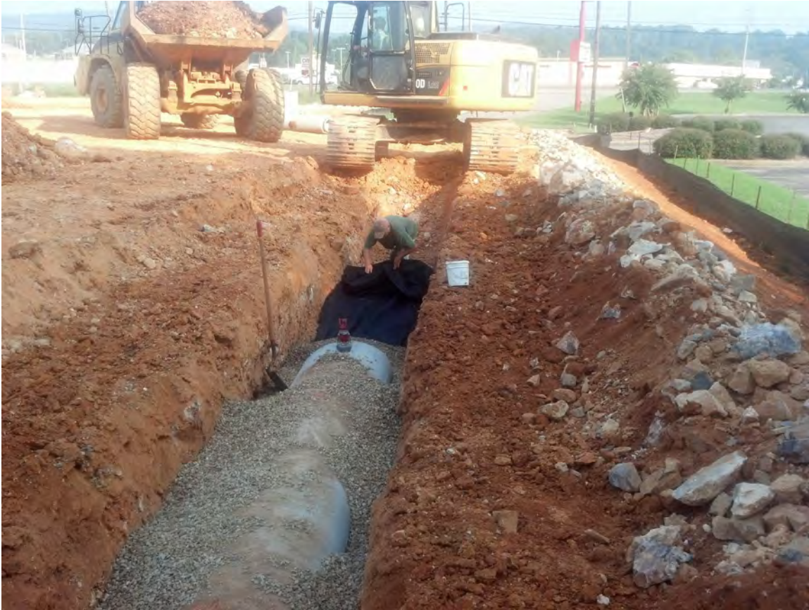
Photo 4: Excavation and placement of piping run over Geotex® 801 nonwoven geotextile marker layer at Station A-2+400.
