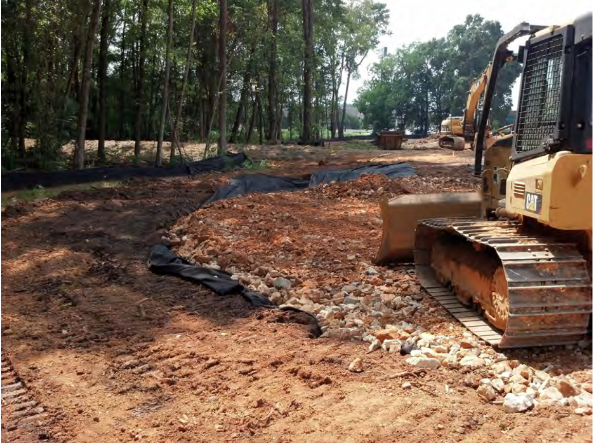
Photo 6: Construction of the roadway turnaround area (Geotex® 801 nonwoven geotextile fabric overlain with gravel following minimal excavation).
