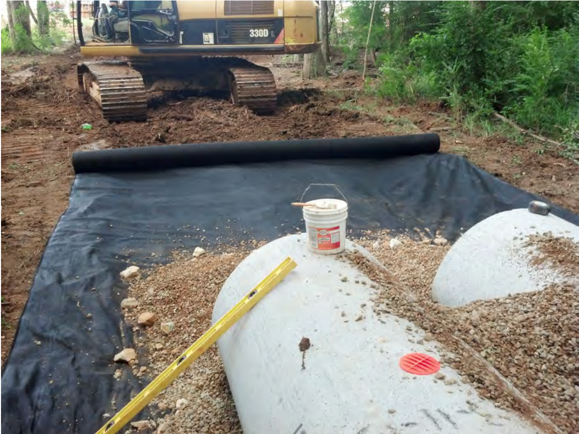
Photo 2: Installation of double piping along Station A-0 to A-2. Geotex® 801 nonwoven geotextile marker layer was overlain with stone and gravel prior to placement of piping.
