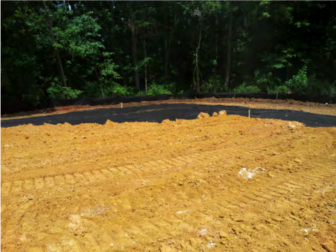
Photo 1: Construction of decontamination pad with Geotex® 801 nonwoven geotextile fabric overlain by clean fill.
