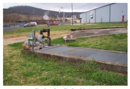
Plant Storm Sewer Pipe Drop Inlet Area
