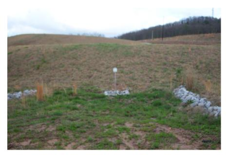
South Landfill Toe Drain and Check Dam
