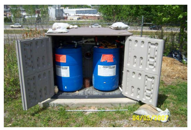
Carbon Treatment Drums in Pre-Fabricated Shed
