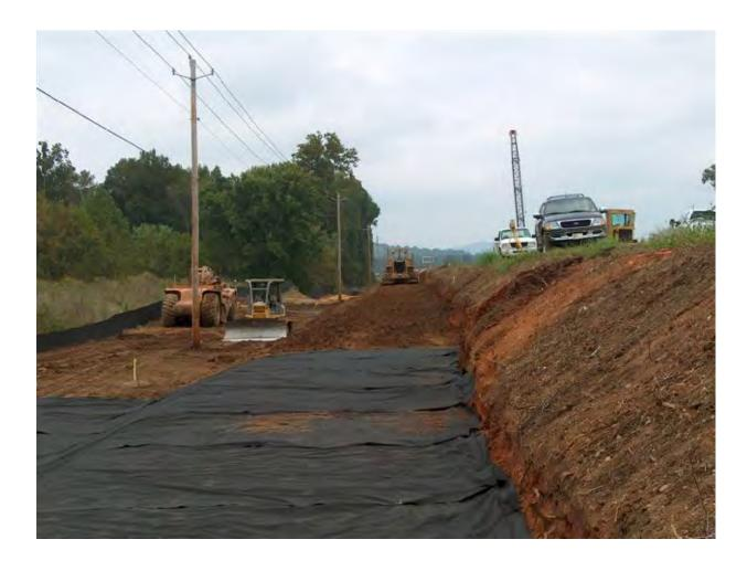
Encapsulated PCB-Containing Soil with Marker Layer
