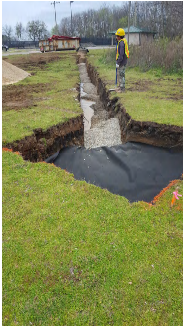
Placement of Marker Layer in Grinder Pump Location and DGA in Sanitary Sewer Connection Trench Prior to Backfilling with Clean Soil Facing Southwest.
