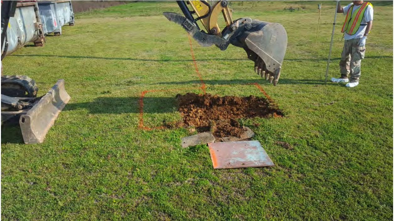
Excavation of Water Service Connection Pit Facing North.
