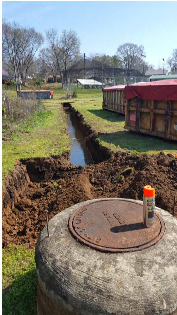
Excavation of Sewer Service Connection Pit and Sanitary Sewer Connection Facing Northeast and Showing Water Intrusion.
