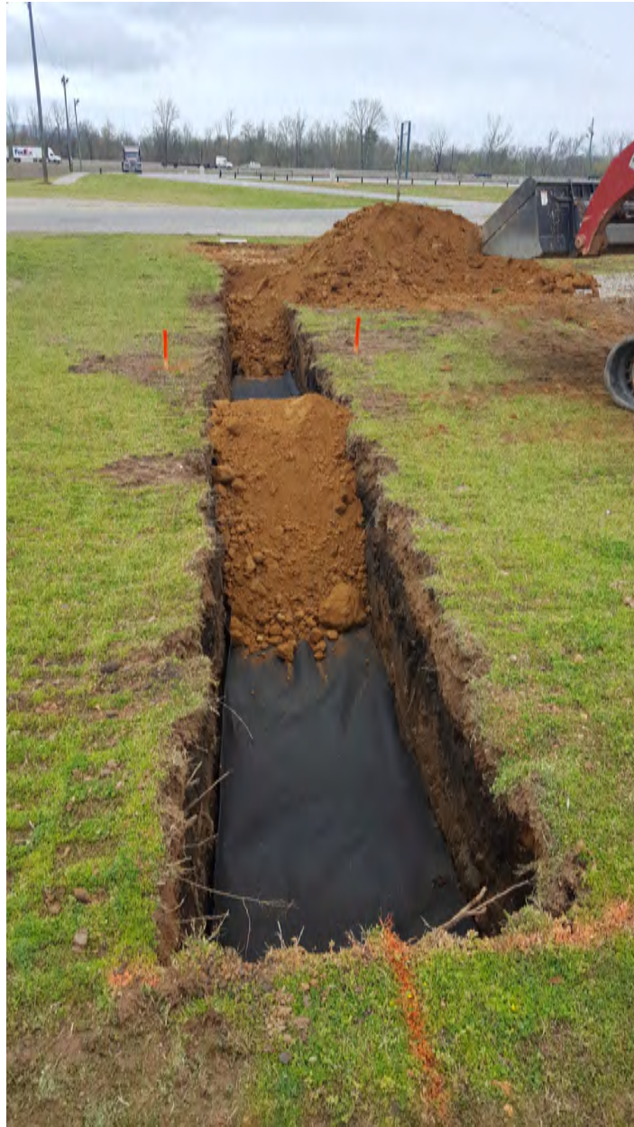
Clean Fill Being Placed Over Marker Layer Facing South.
