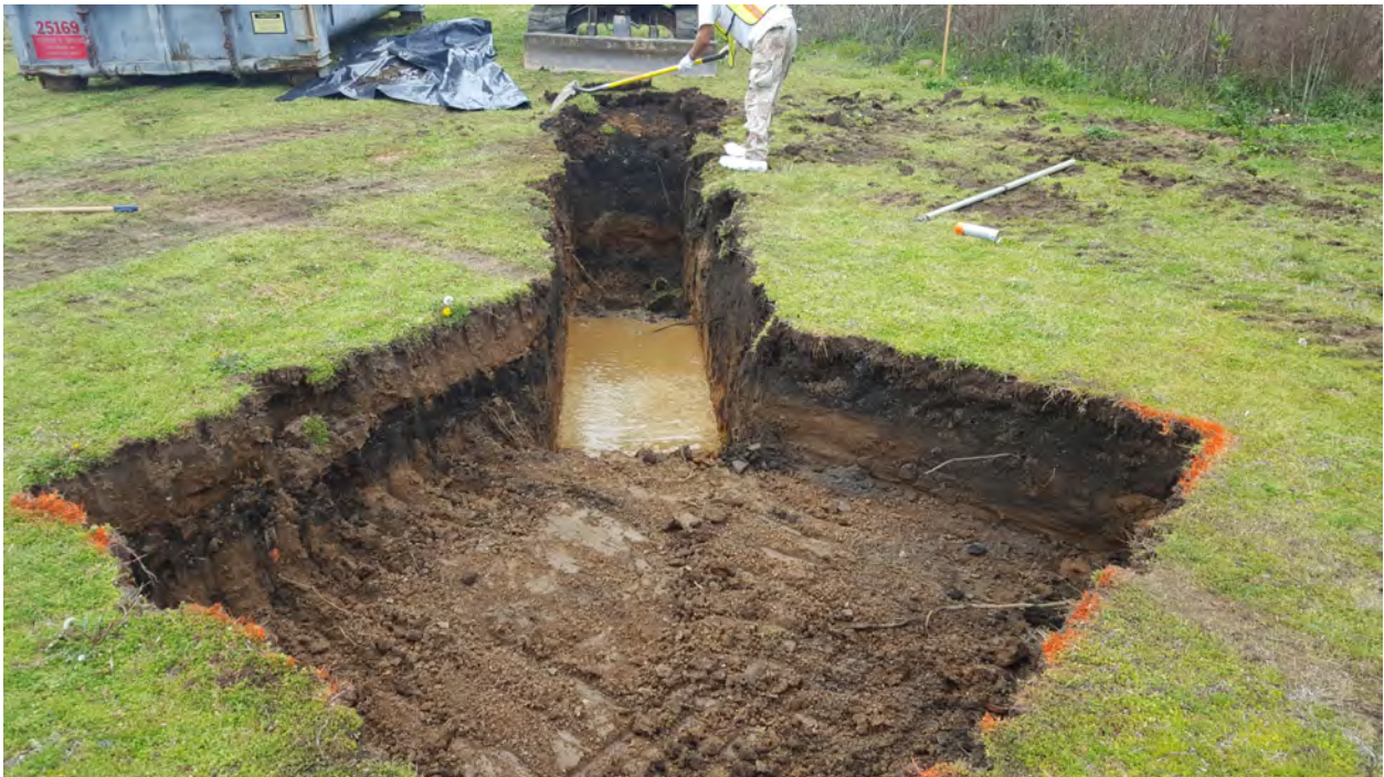
Excavation of Grinder Pump Location Facing Southwest Showing Water Intrusion.
