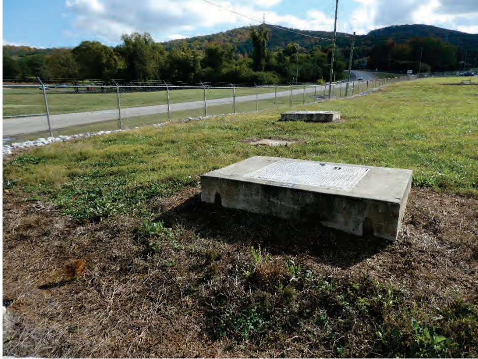
Vaults for interceptor wells near CTS #2
