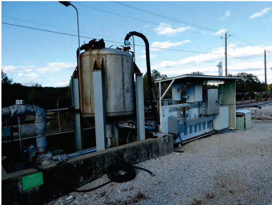
Temporary storage tank for WMA II corrective action system and CTS #1 to treat extracted groundwater in the vicinity of OW-21A
