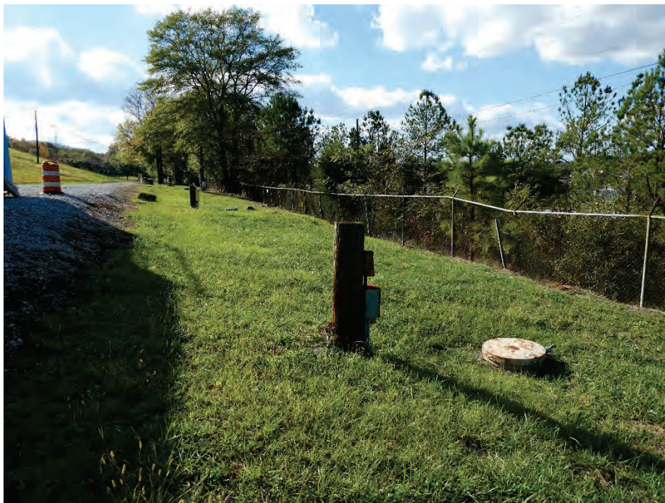
Line of extraction wells north of the South Landfill
