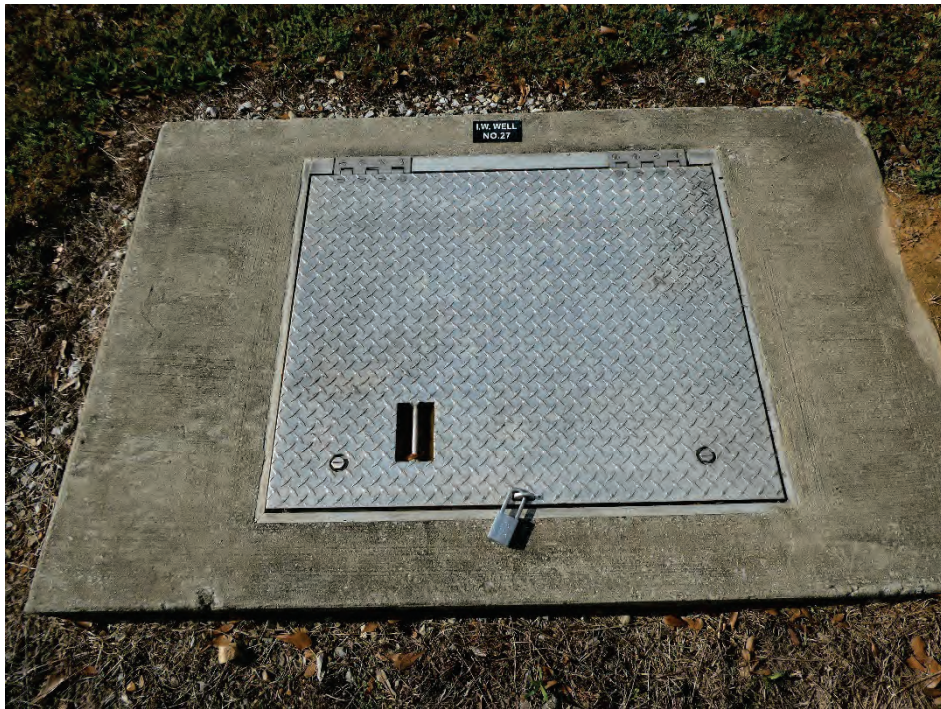
Locked vault for interceptor well 27
