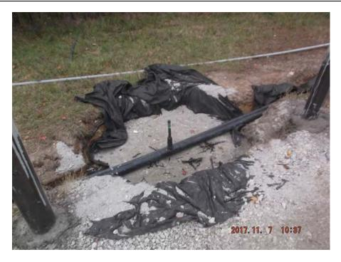
(2) Combination air valves were installed on CTS#3 effluent piping (3" diameter SDR 11 HDPE) at high system locations as indicated in the design specifications.
