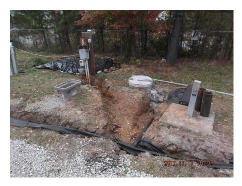
(1) Installation of conveyance piping (2" diameter SDR 11 HDPE) for intercept (IW) wells, and Carbon System No. 3 (CTS#3) effluent piping (3" diameter SDR 11 HDPE) began on 19 October 2017.
