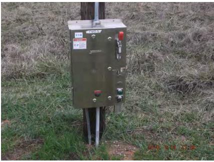
(1) IW well upgrades, including installation of new downhole pumps (Grundfos), and extraction system piping, were completed between January and February 2018. New electrical control boxes and instrumentation were installed at the IW wells.
