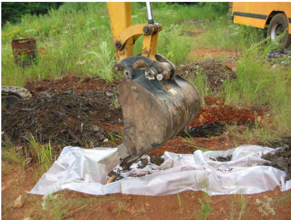
Photograph 2 – Excavating through cover soils into auto fluff debris.
