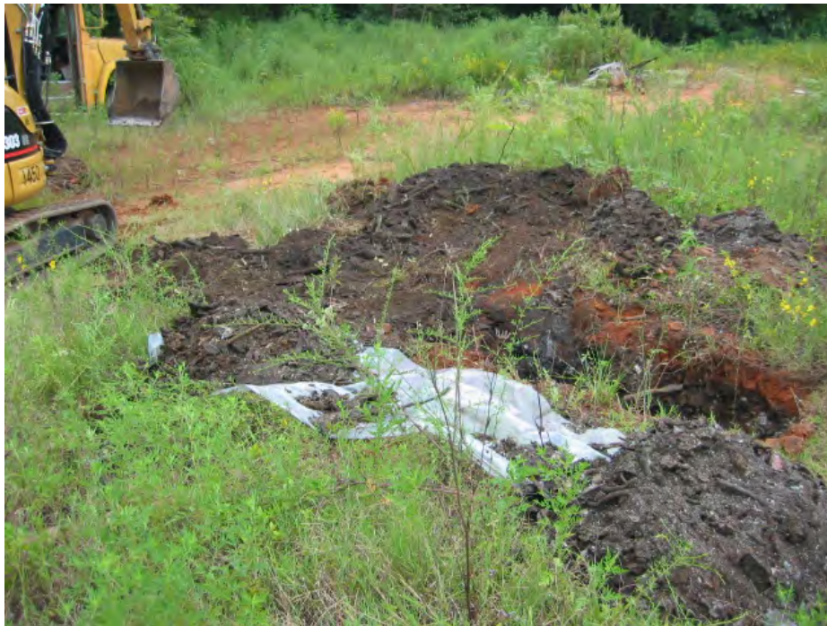
Photograph 1 – Test pit excavation showing auto fluff debris and reddish cover soils.
