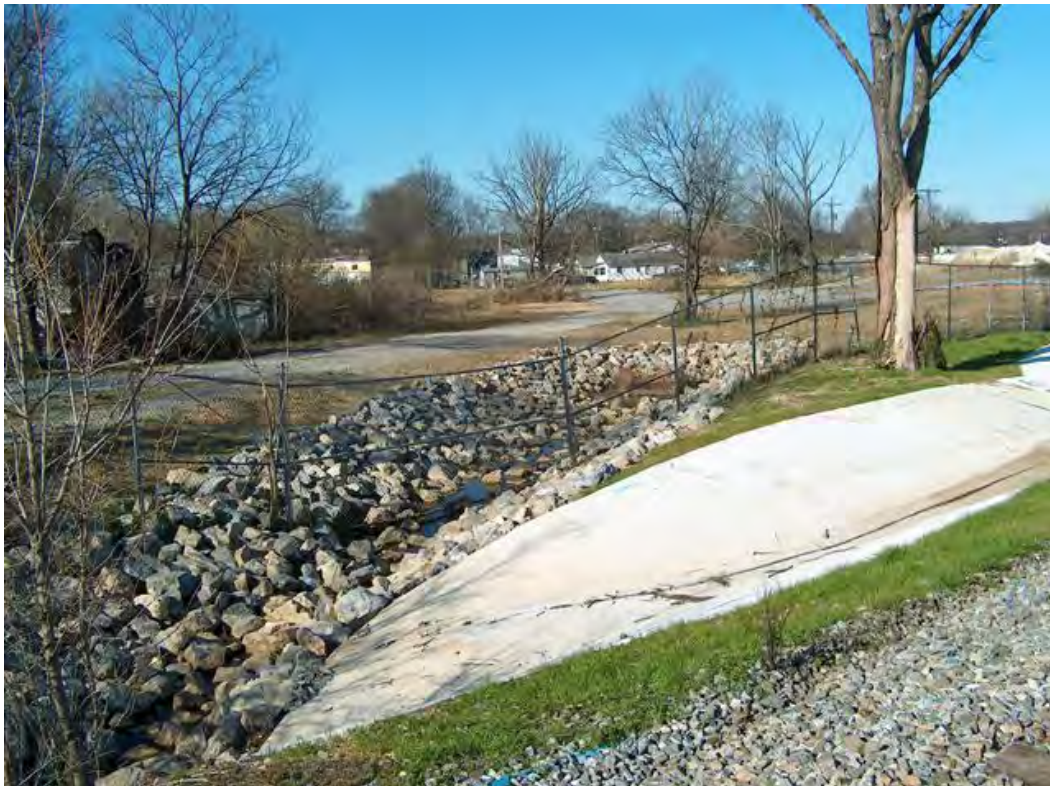
Rip rap area within vegetated swale north of ditch segment B4. Photo looks north.
