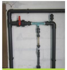
When there is no injection pump available, the product can be incorporated into the water by suction through a Venturi system
