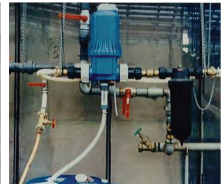
Alternatively, a pump can be connected directly to the drum containing metam (most common method).
